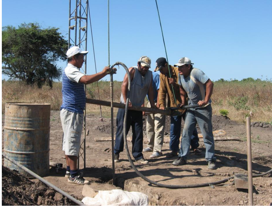
Figure 3-9. EMAS percussion-jetting-rotation manual drilling, Trinidad (Beni region)
